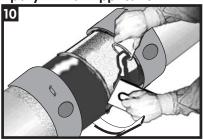
Apply mixed epoxy to a uniform specified thickness of 4-6 mils (100-150 microns) on all exposed bare metal using the applicator pads as supplied or an approved tool. Do not apply the epoxy to the mainline coating. Use a wet film thickness gauge to confirm the thickness.
