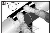
Place the underlap of the sleeve onto the joint, centering the sleeve such that the sleeve overlap is positioned at either the 10 or 2 o'clock position. Ensure that the sleeve is placed square to the pipe.
