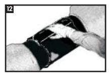
Press the closure firmly into place. Ensure the closure is in complete contact with the underlying sleeve.
