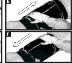
Gently heat the closure and pat it down with a gloved hand. Repeating this procedure, move from one side to the other. Smooth any wrinkles by gently working them outward from the centre of the closure with a gloved hand.
