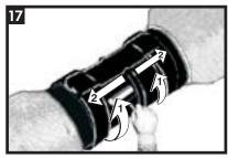
While the sleeve is still hot and soft, use a hand roller to gently roll the sleeve surface and push any trapped air up and out of the sleeve, as shown above. If necessary,
